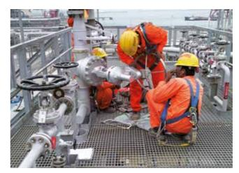
Netherlocks guarantees at least 10 years lifetime of the valve interlock and this is backed by TUV testing and certification. The simple and reliable mechanical design has proven itself over 20 years in the field.
